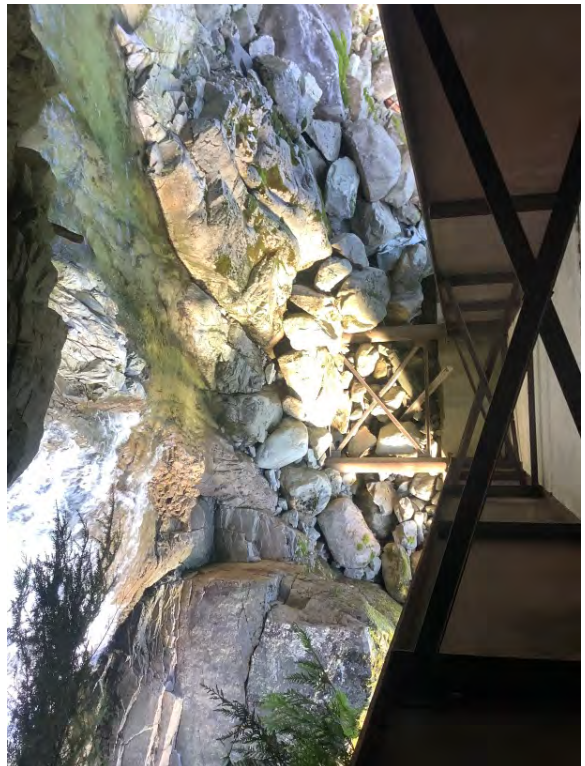
Left Bank Abutment when facing downstream
