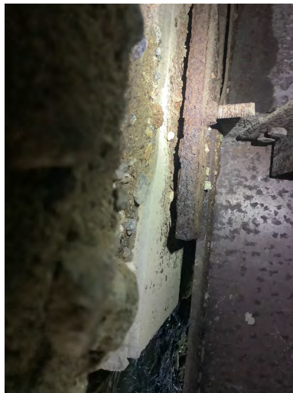
Right Bank Abutment when facing downstream - us inside bolt
