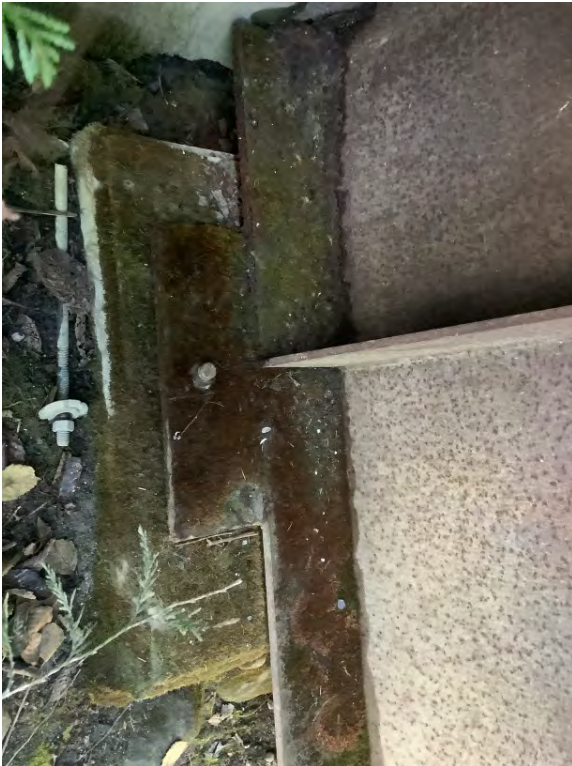
Right Bank Abutment when facing downstream s DS
