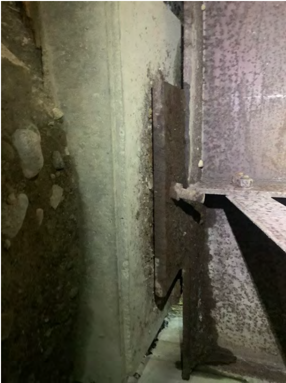
Right Bank Abutment when facing downstream - DS inside bolt
