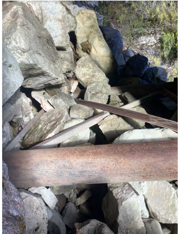
Left Bank Abutment when facing downstream
