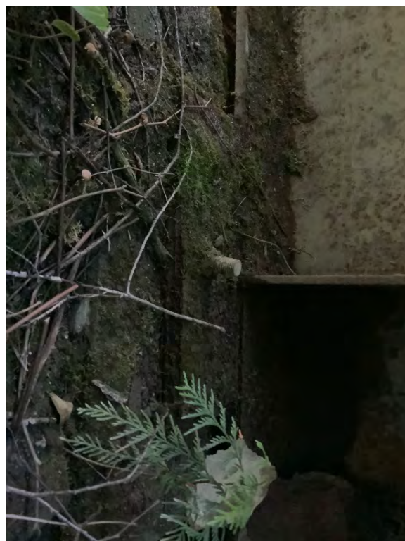
Right Bank Abutment when facing downstream - us outside bolt
