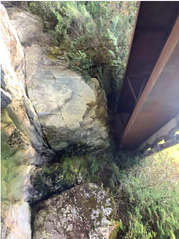
Right Bank Abutment when facing downstream
